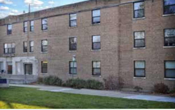
This example shows Lamson Hall retrofitted with a securable archway to access the northern courtyard.
